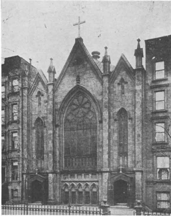
Exterior of the Old Church
